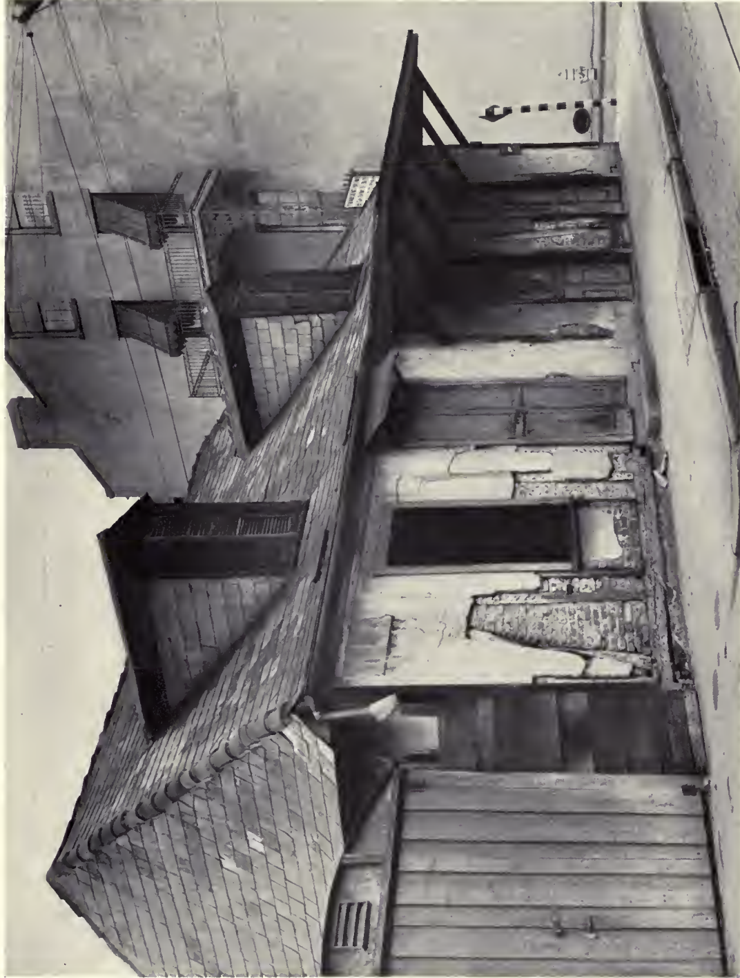
Typical "Brique de Poteux" Construction Measured Drawings, 118 and 119
